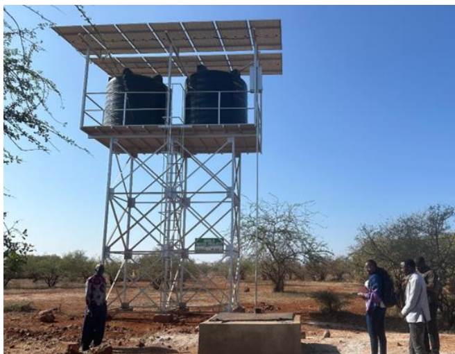
Figure 7: A solar-powered borehole in Moilo Primary that serves the school and the neighbouring village.
